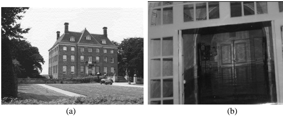
Figure 2: (a) Amerongen Castle and (b) the entire basement of the building was flooded twice from the nearby Lower Rhine river in 1993 and 1996
